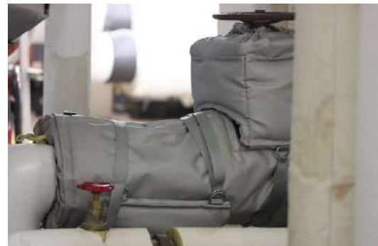
Removable Insulation Blankets
