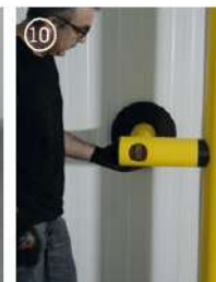
Ensamblaje brazo a pared/panel Assembling the arm to the wall/panel
